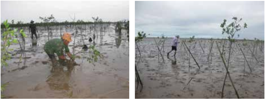
Figure A7: Planting and piling
