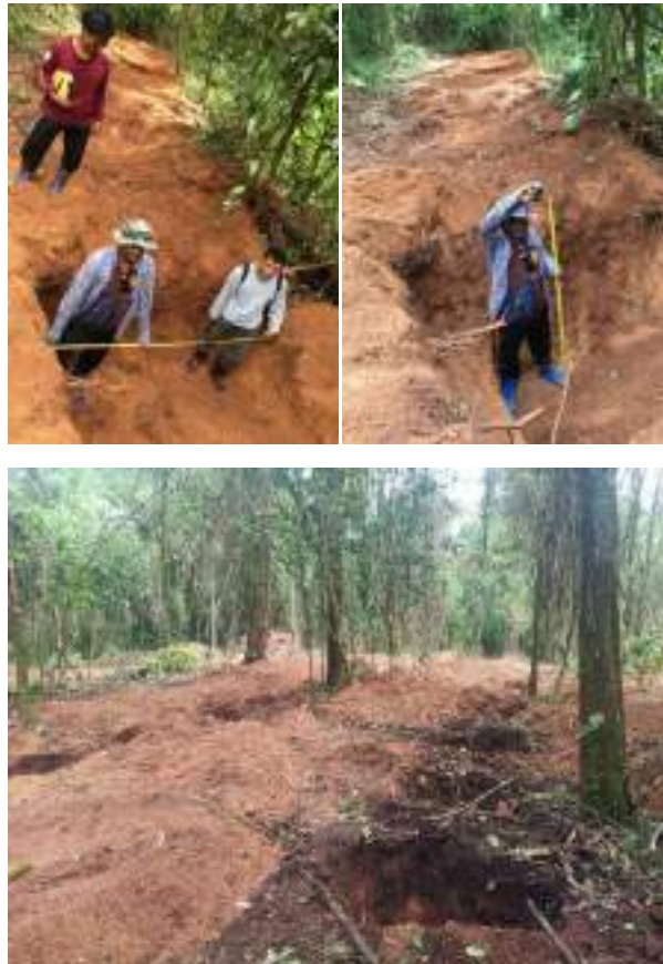
Figure 2 a,b) Checking hole size after Caterpillar dig a hole c) Hole planting line
