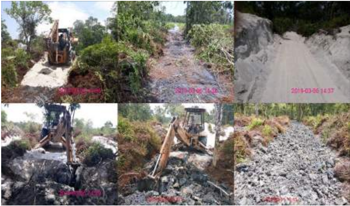
Site preparation of 2019 planting
