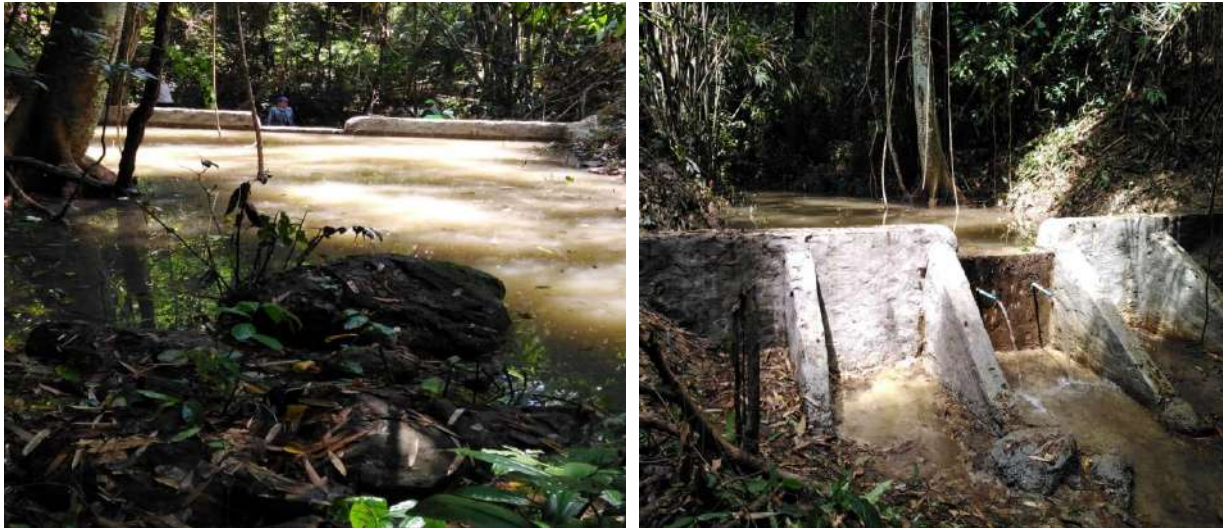
Figure 13. A small check dam in Phoukhanya mountain can store water
