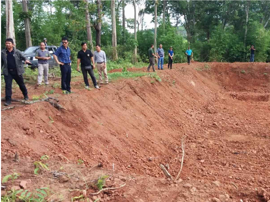
Photo 4: Water pond under construction in Loei, Thailand
