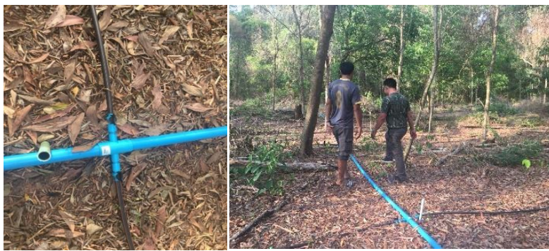
Figure 9: Irrigation system maintenance (fix change ,repairing).
