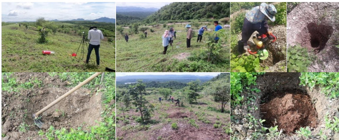
Figure 7: Site preparation of Mae Moh plot.
